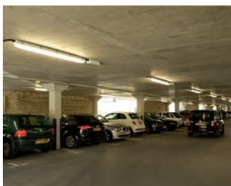
White Rose Office Centre Car Park | 44
