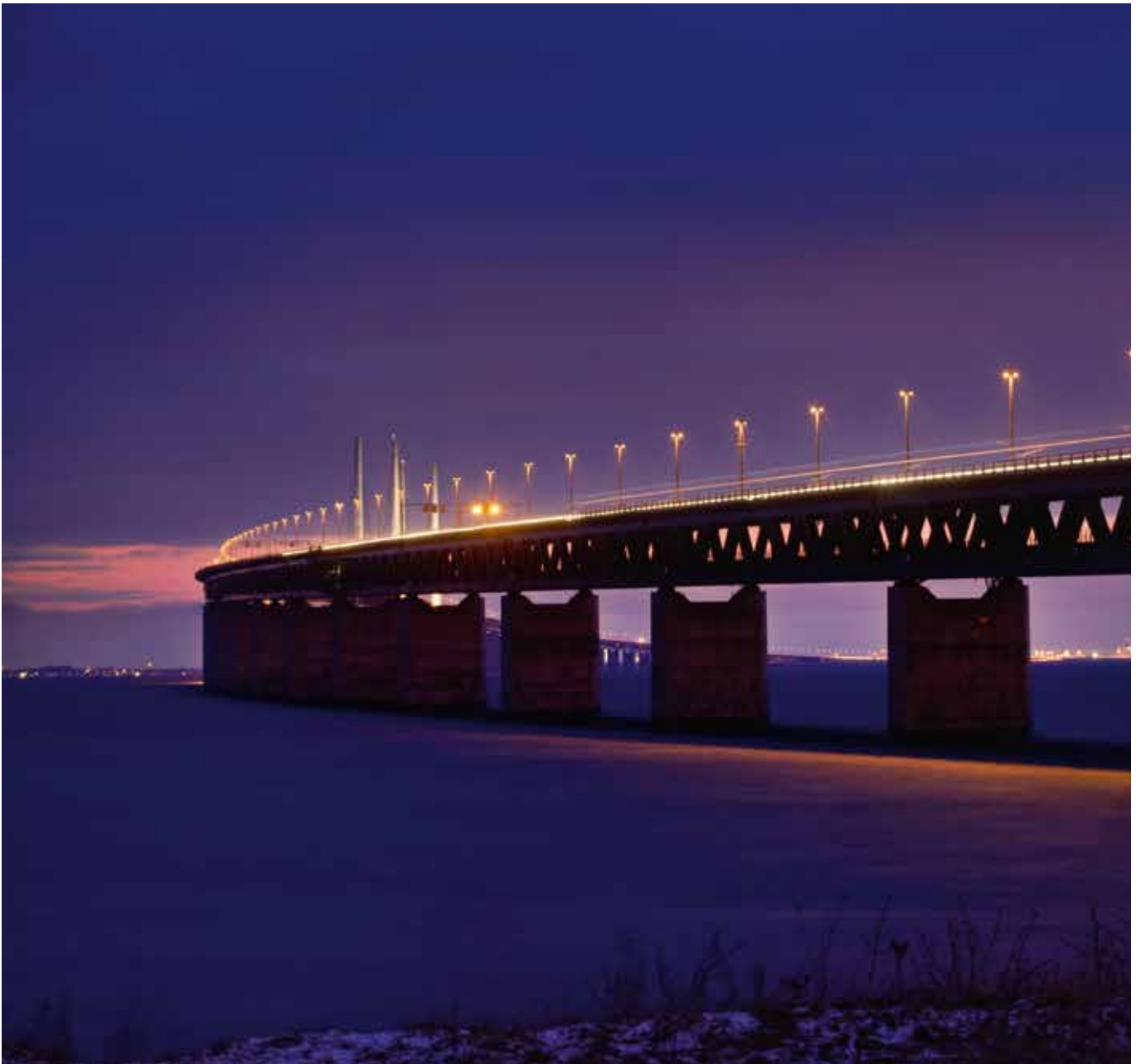
Øresund Bridge, Copenhagen, Denmark
