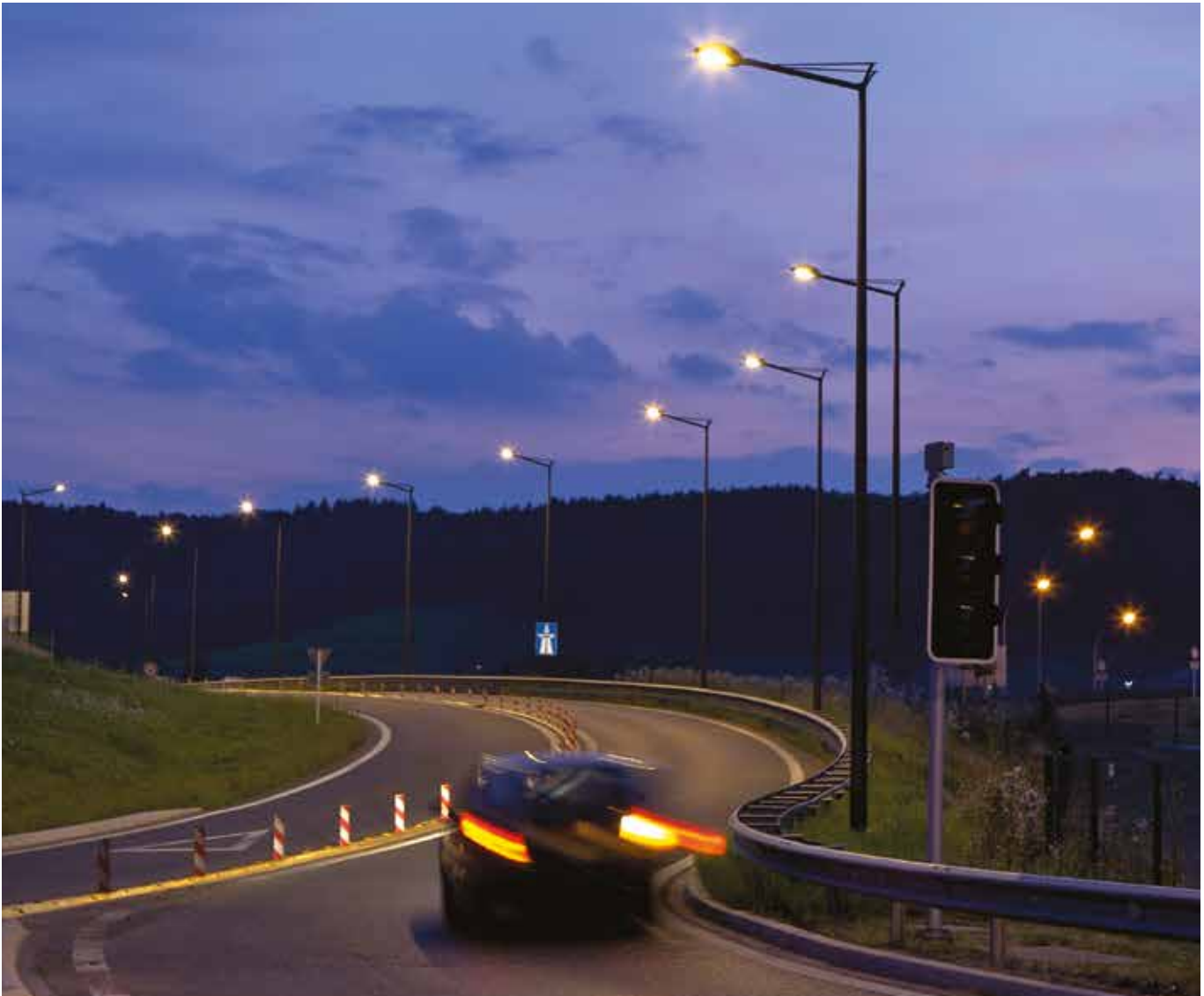
Norrtsleden Highway, Stockholm, Sweden
