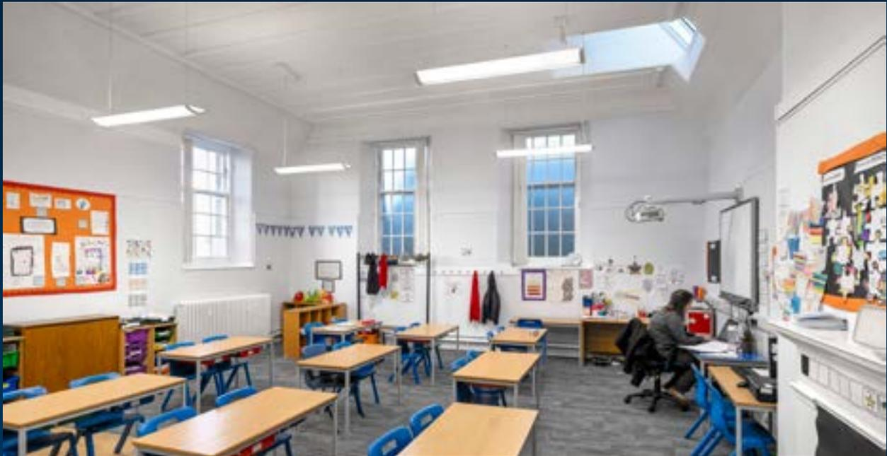
various tasks, the general space and the different forms of personal communication between teachers and pupils. A range of integrated control systems such as daylight, presence and absence detectors with PIR and microwave sensors, support further energy savings and empower users to manage their own lighting scenes. IQ Wave achieves a unified glare rating of <math><19</math>, in line with the EN 12464 standard on workplace lighting.
