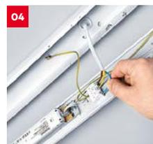
04 Connect power cable to terminal block
