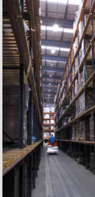
50% saving as worker activates lights and stops half way down
