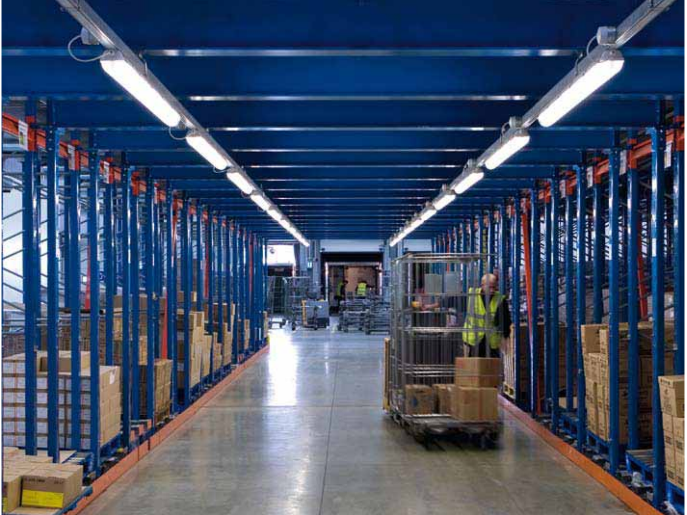
ImpactForce has been fitted in the storage and racking areas because of its robust construction and resistance to impact and vibrations.
